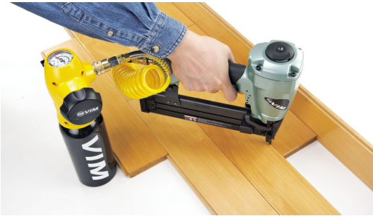
Wood Floor Nailing
