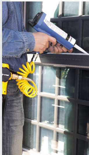
Window, Door, Bathroom Caulking
